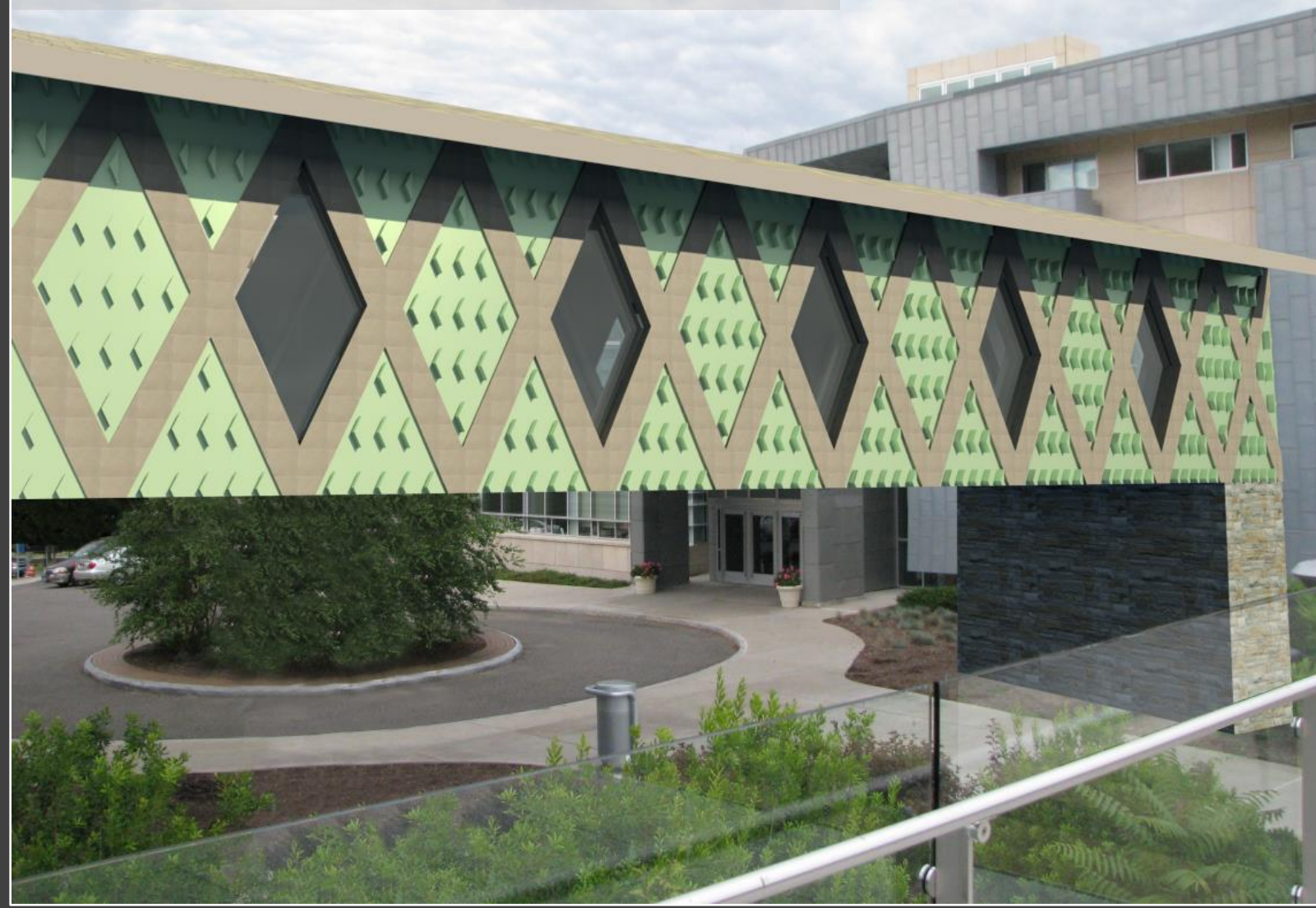
Redesigned Bridge Façade
