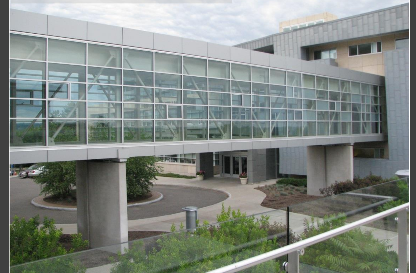
Existing Bridge Façade
